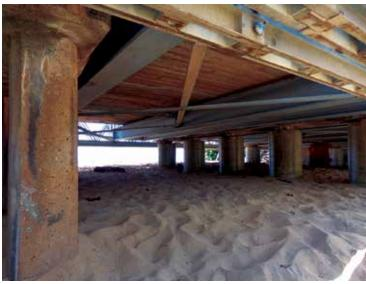
When a state inspection found serious deterioration in the support piers of the 87-year old Paumalu Stream Bridge's support piers, a plan for expedited repairs was undertaken in order to avoid further structural damage. Although the heavily used bridge was repaired as recently as 2014, it was decided to again renovate rather than replace the structure in order to minimize the impact on the public.
