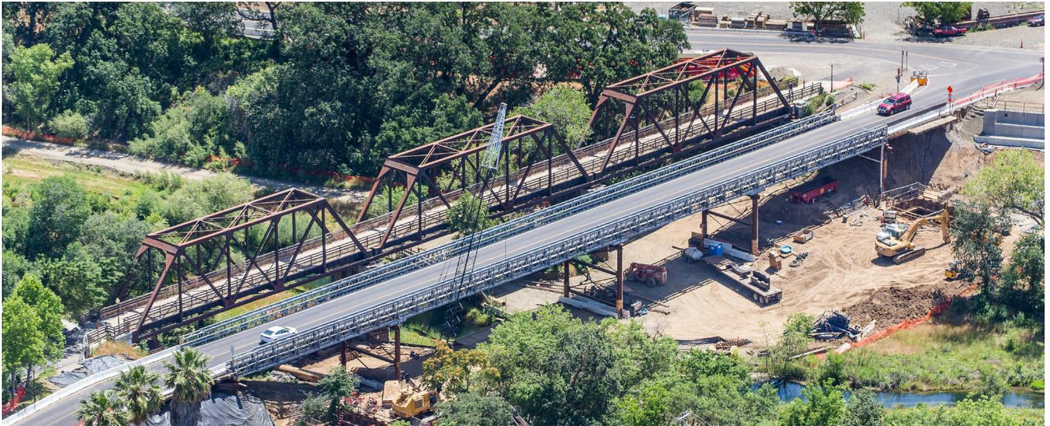
Originally built in 1908, the Winters Road Bridge arches over the Putah Creek, connecting Yolo and Solano counties. In 2007, this historic bridge received the lowest safety rating among Solano County-owned bridges due to water damage on the exposed timber pilings under the bridge's pier supports. The damage to the structure's foundation was determined to be irreparable.
