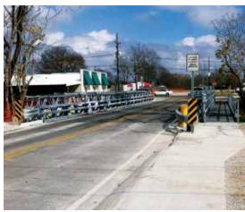
With deteriorating timber piles, two old bridges in Terrebonne Parish were failing and could no longer handle even typical vehicular traffic. Terrebonne Parish Consolidated Government purchased two modular steel bridges from Acrow to replace the critically deficient structures in Houma and Gibson. Acrow's prefabricated panel bridges provided a simple design, reduced installation time and overall project cost benefits, while meeting and exceeding the load and design requirements.
