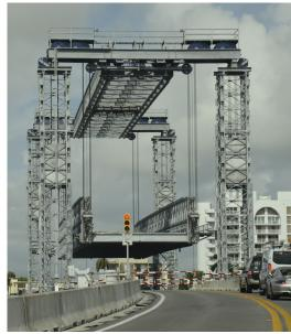
Connecting the Town of Palm Beach and the City of West Palm Beach, the Southern Boulevard Bridge is one of three bascule bridges crossing the Intracoastal Waterway and Lake Worth Lagoon. When structural problems were found with the bridge, it was determined that a temporary lift span would also be needed during the replacement process to accommodate heavy vehicle traffic on the roadway as well as commercial and recreational vessel travel in the waterway below.
