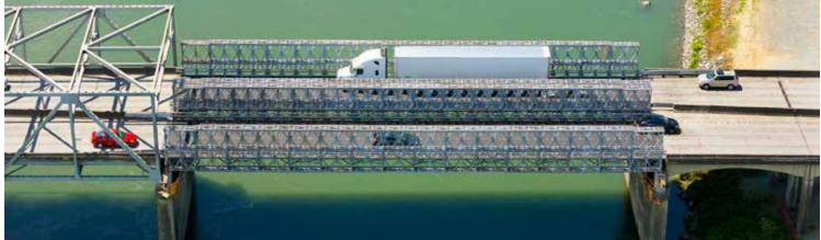
After the collapse of the I-5 Bridge over the Skagit River in Burlington, WA, the WSDOT had to find a quick and safe solution to solving a financial disaster in the making. In conjunction with Atkinson Construction and the WSDOT, an Acrow 700 XS panel bridge was commandeered as an emergency temporary bridge over the Skagit River.
