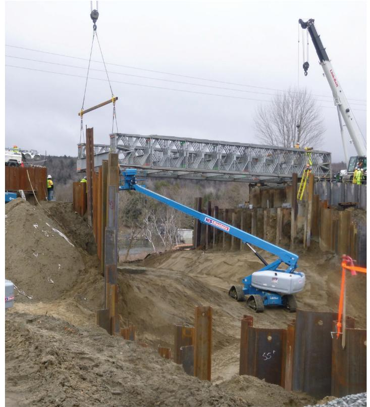
Hydraulically undersized and failure-prone, then further damaged by Hurricane Irene in 2011, the Manchester Brook culverts under US Route 5 and the Washington County Railroad (WACR) were contracted for replacement using the design-build project delivery method. Vermont Agency of Transportation authorized the team of Dubois & King (designers) and Engineers Construction Inc. (ECI) to proceed with the \$15.2 million project in May 2014.
