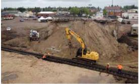
In late June 2015, an overpass on U.S. Route 85 in Lusk, Wyoming collapsed onto railroad tracks as a result of heavy rains and flooding of the nearby Niobrara River. The collapse created an immediate stop to the passage of daily Union Pacific Railroad freight trains, up to 12 coal trains per day, as well as vehicular traffic on Route 85.
