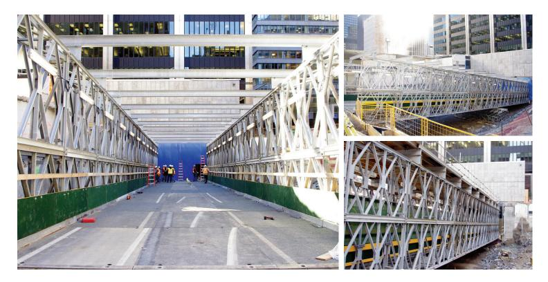
Acrow supplied PCL Constructors Canada with a prefabricated modular steel bridge that spans an excavation site at PCL's 100 Adelaide Street West Project in downtown Toronto. Serving as a temporary ramp, the 36-meter bridge was designed to provide delivery trucks and other vehicles with secure access to loading docks that serve a number of buildings, restaurants, and businesses in the vicinity. The Acrow ramp will provide access for 18 months, while a new 43-storey office building is constructed.
